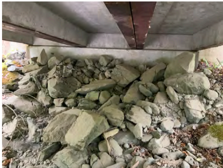
Right Bank Abutment when facing downstream
