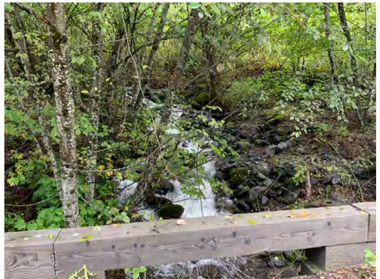
Upstream from Crossing
