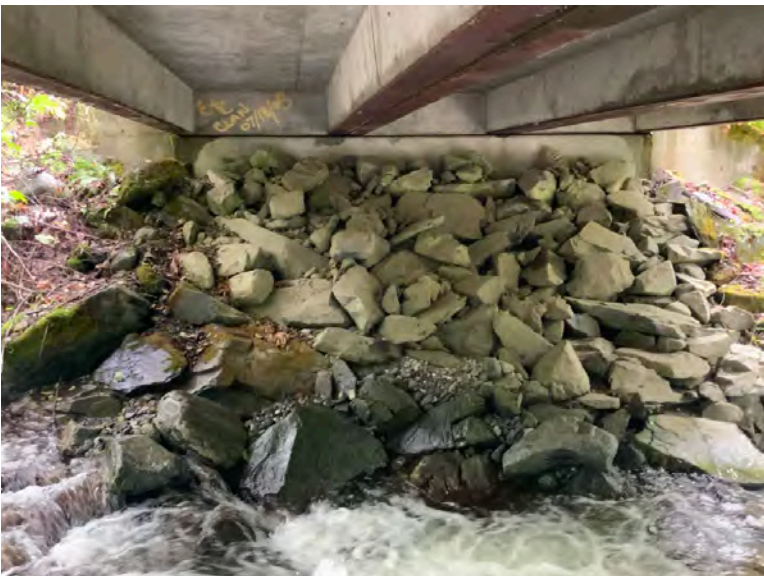
Left Bank Abutment when facing downstream
